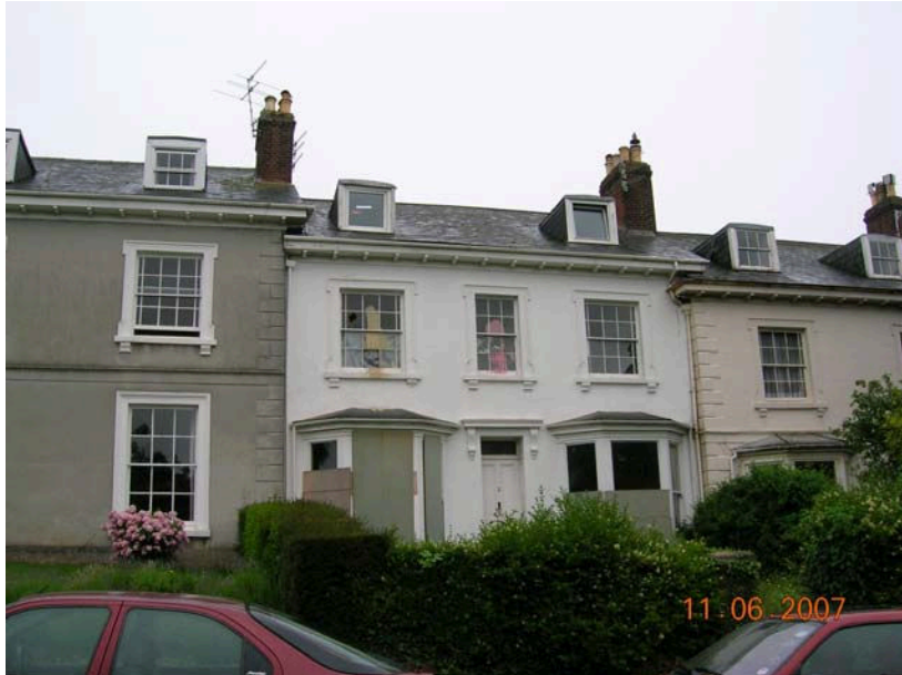
Exterior after squatters had damaged the building in 2007
